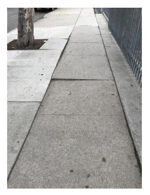
Tree roots lifting sidewalk can cause a difficult walking environment on East 78th Street
