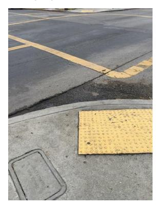
Curb ramp in the northeast corner of the intersection East 79th Street and McKinley Avenue has possible ponding, degraded pavement, and vertical grade differences over one-half inch
