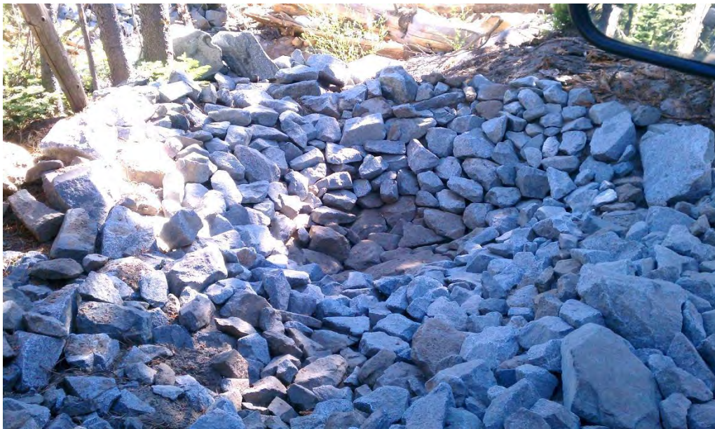
Rock lined outlet protection with sediment trap
