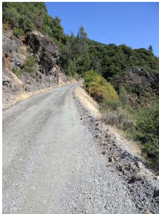
Outside shoulder with additional windrowed material for future needs and safety
