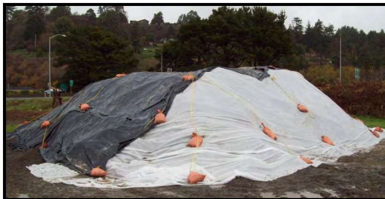
Proper securing of plastic sheeting.
