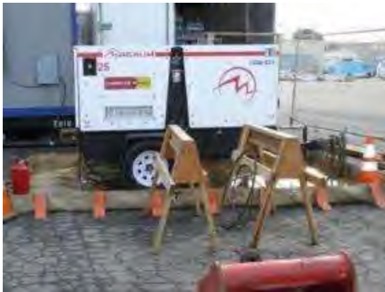
Generator on secondary containment
