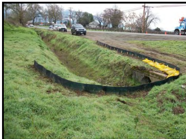
Silt fence reinforced with gravel bags.
