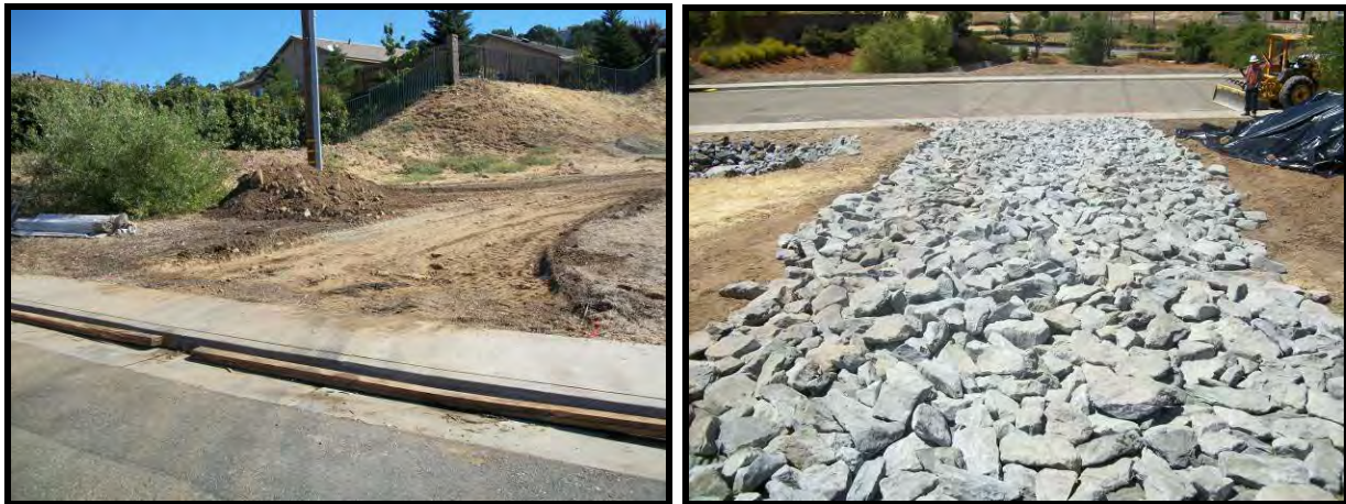
Construction entrance/exit before and after installation.
