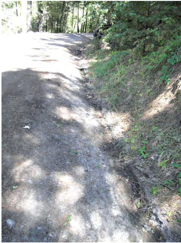
Cleared ditch without undercutting uphill slope
