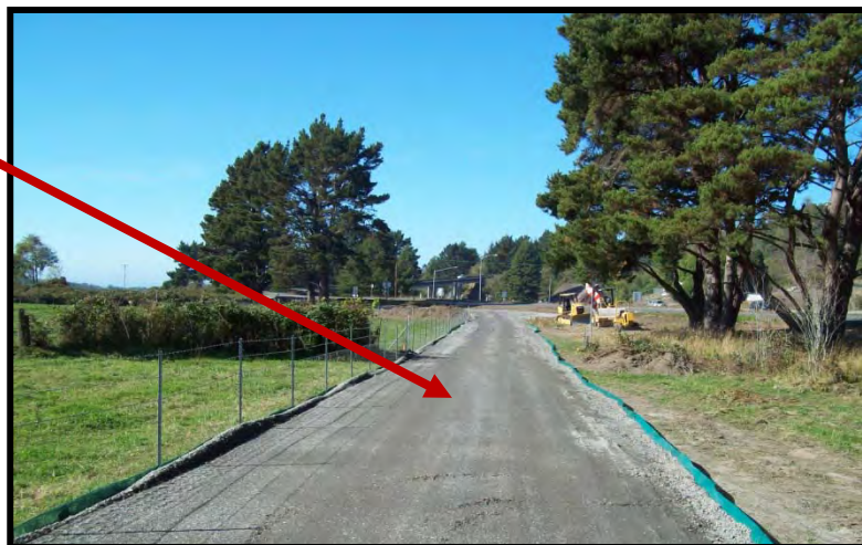
Stabilized construction road.
