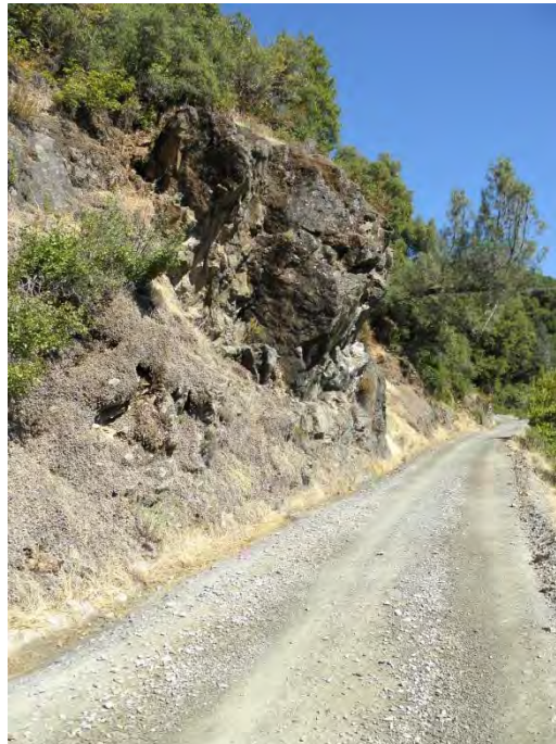
This dry road still looks wet, and remains dust free several weeks after application of chemical dust suppressant.
