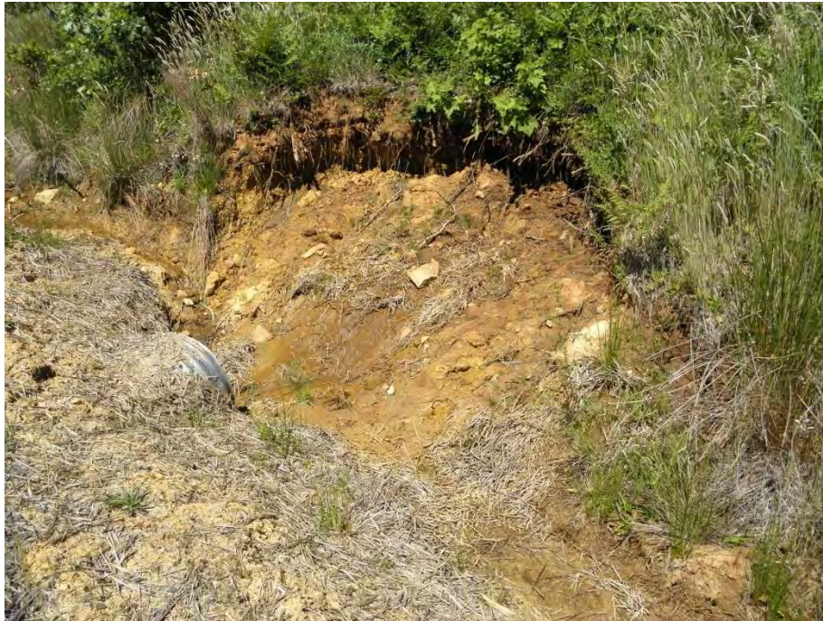
Slide material removed from culvert entrance
