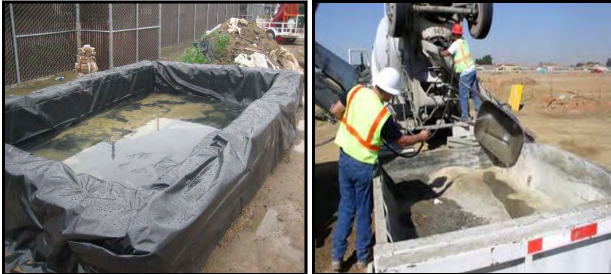
Two alternatives for containing concrete washout water.
