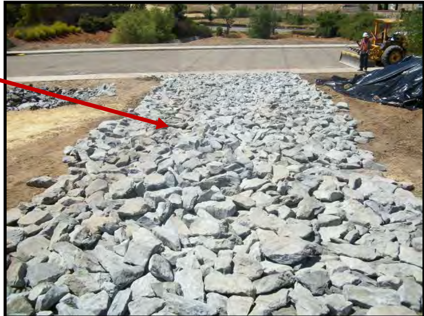
Traditional rocked construction entrance/exit.
