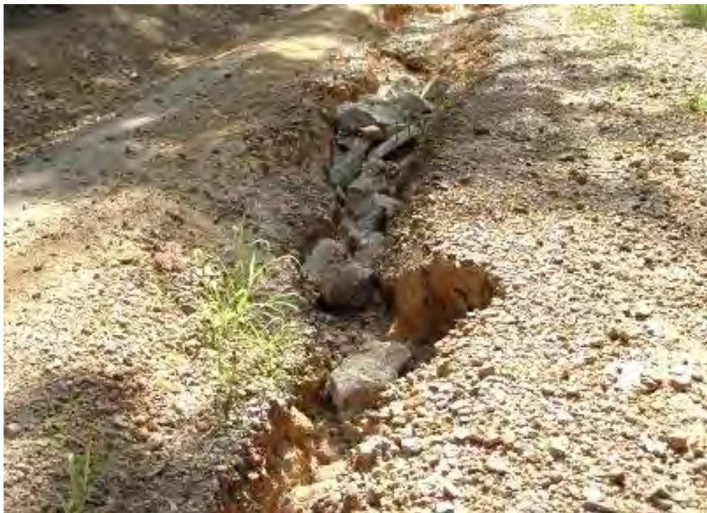
Gullies must be filled with suitable materials to prevent re-occurrence and expansion.
