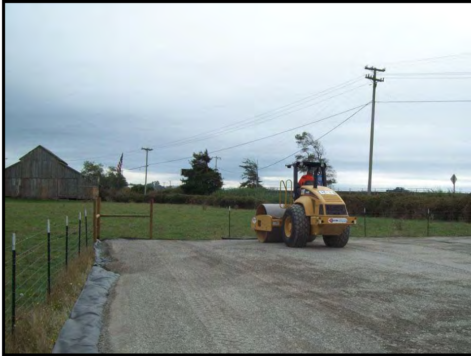
Gravel stabilization being installed.
