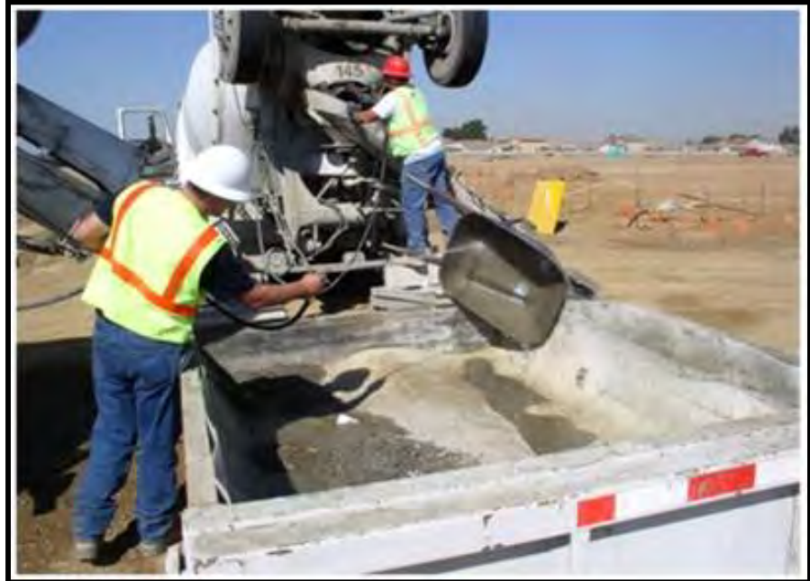
Self contained concrete washout.
