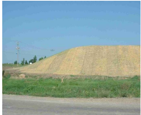
Figure 4. Stockpile stabilized with erosion control blanket
