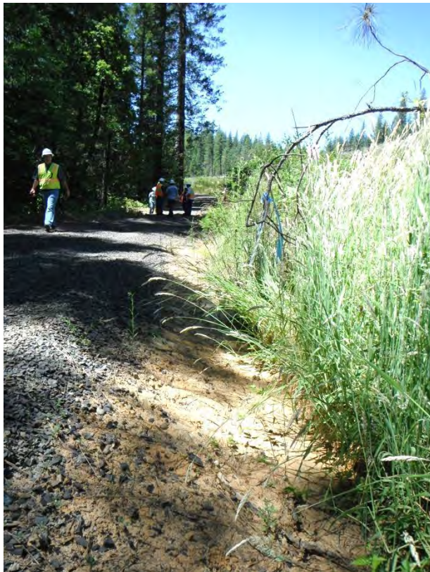
Native grasses left on uphill slope to dissipate energy coming off of slope.
