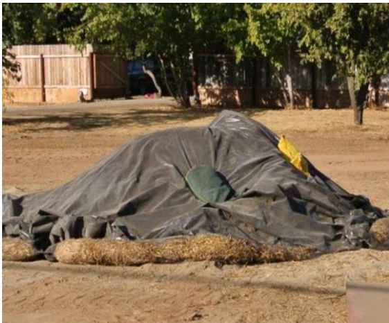
Figure 5. Contaminated stockpile under cover
