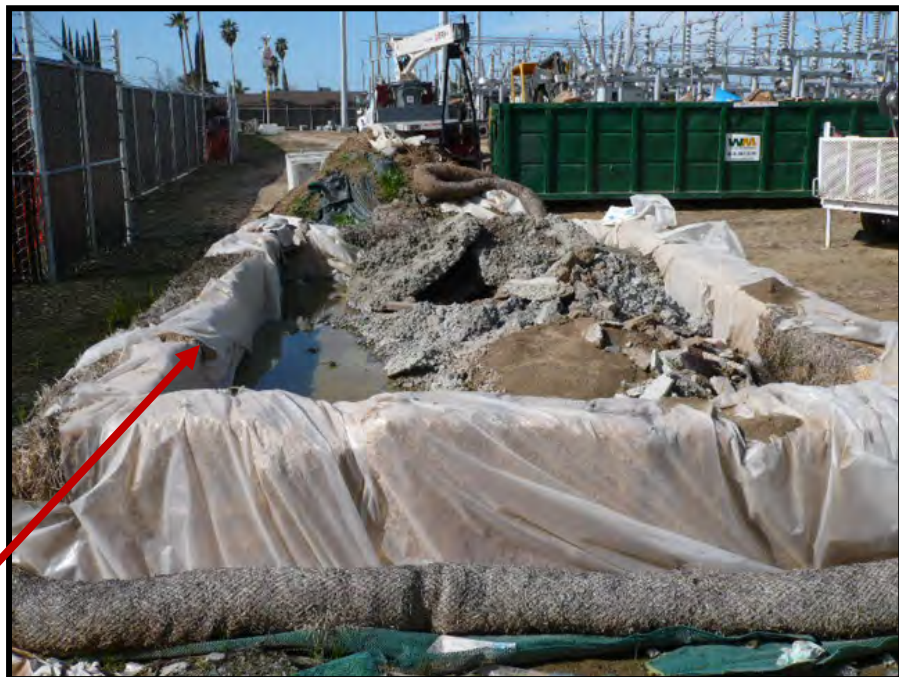
Lined concrete washout.
