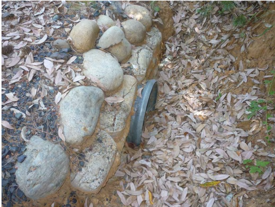
Replaced culvert with dry stacked concrete bag headwall
