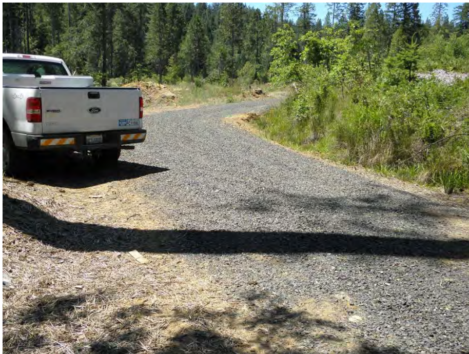
Imported Material Bladed Access Road
