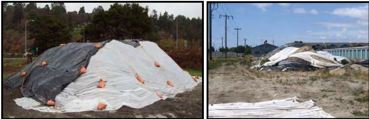
Plastic sheeting over stockpiles properly and improperly secured.
