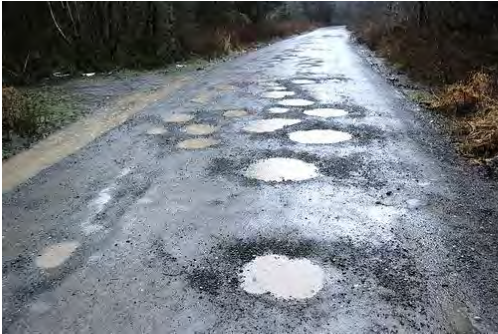
Road surface after several weeks of heavy rain and repeated use.
