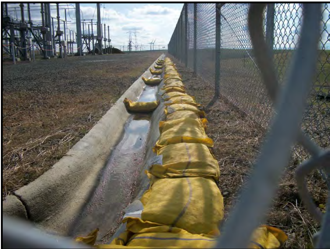
Gravel bags used to slow sheet flow run-on into the lined swale, and as check dams to slow flow within the swale.
