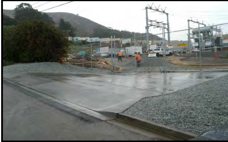
Clean and well maintained construction entrance/exit.
