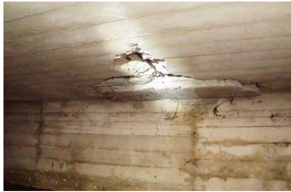
FIGURE 17: Spalling of interior concrete in the channel
