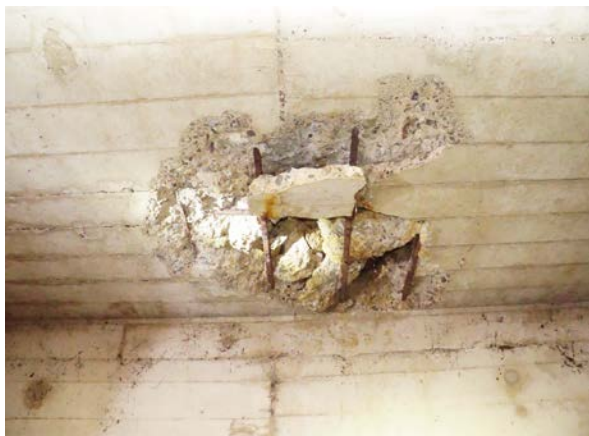
FIGURE 19: More concrete channel spalling
