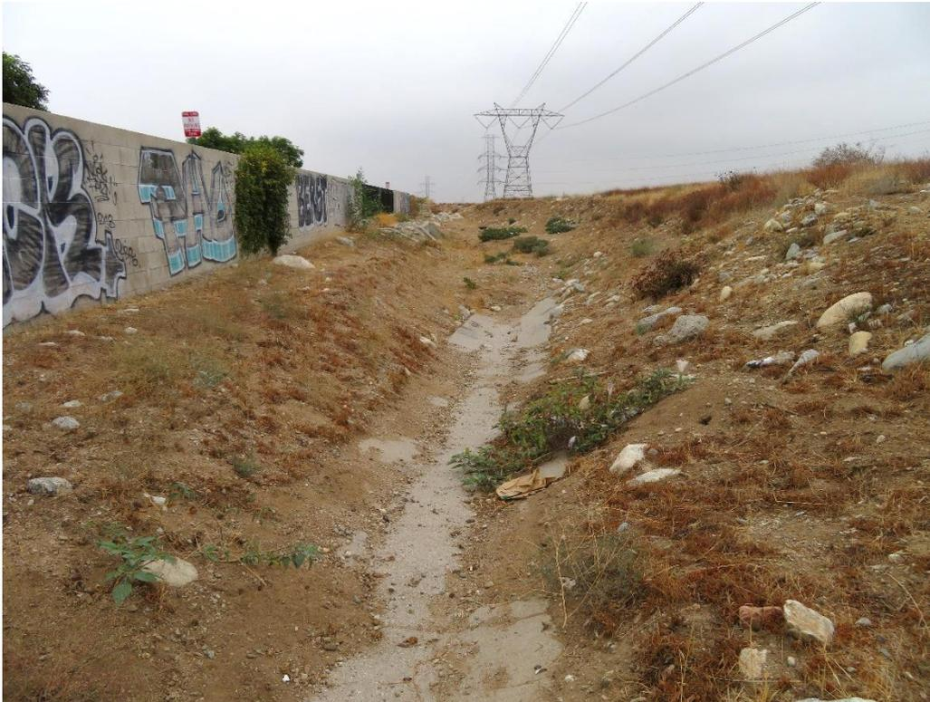
**Photograph 3:** View of the 2-foot concrete lined v-ditch portion of Drainage 1 located along the eastern boundary of the project site.
