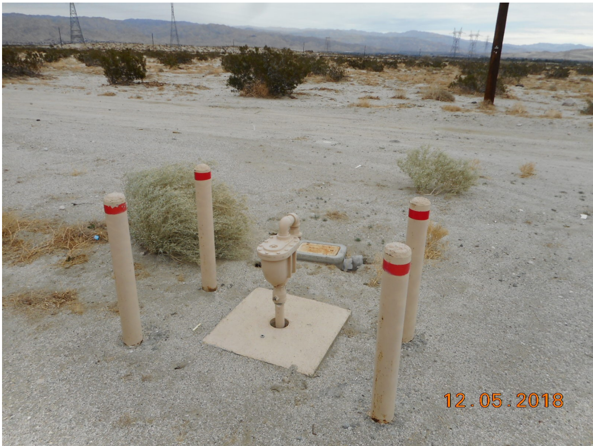
Photo 23 - The four crash posts and apparent water line related piping shown here are located several hundred feet south of the Well No. 33 fenced compound along the west side of Little Morongo Road. Within the dirt road along Little Morongo Road, just above the center of the photograph, is a manhole cover associated with a Mission Springs Water District underground water line.
