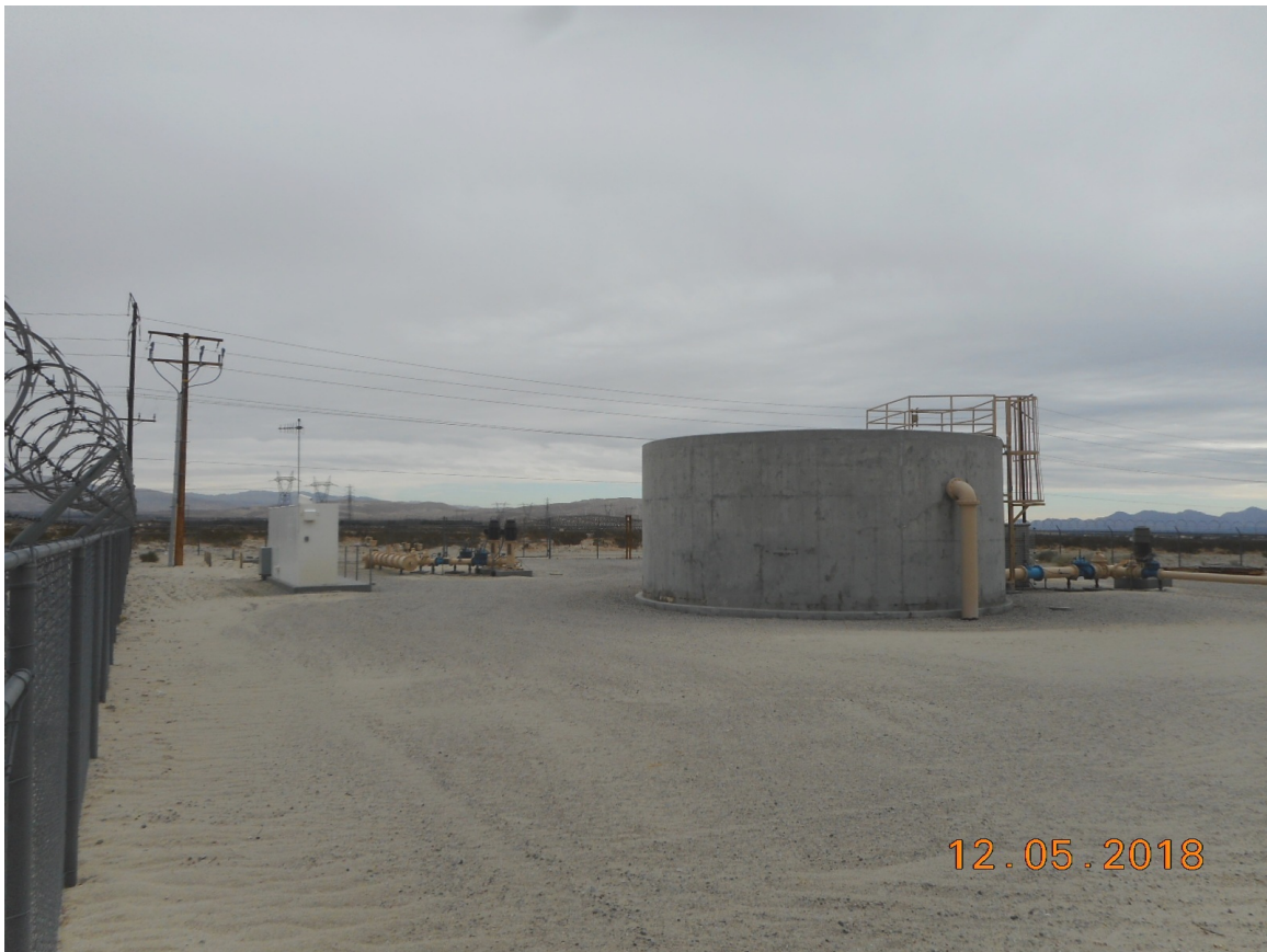
Photo 13 - Easterly view from the northwest corner of the Well No. 33 fenced compound. The white structure to the left houses the electric panels for the Well No. 33 pump and booster pumps.
