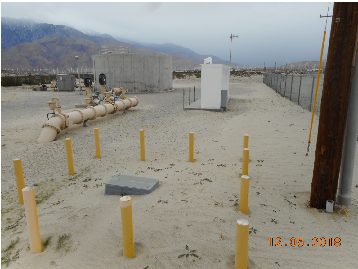
Photo 15 - Westerly view from the northeast corner of the Well No. 33 fenced compound. The piping in the foreground to the left includes connections to two booster pumps with availability for two more booster pumps.
