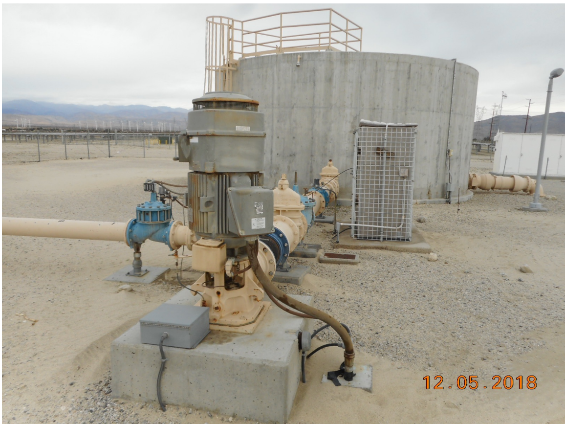
Photo 18 - Northerly view showing Well No. 33 with the suction reservoir beyond. Well 33 is set up to extract groundwater around 900 gallons per minute.
