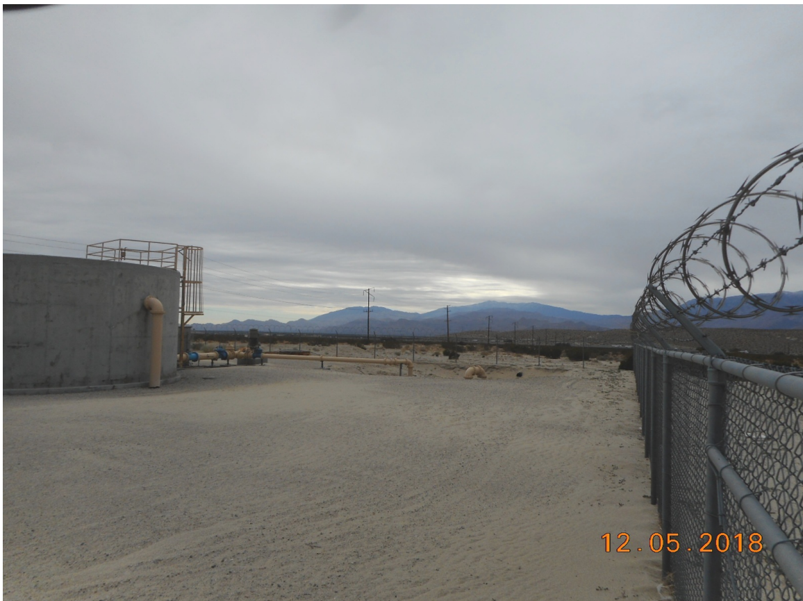
Photo 14 - Southerly view to the right of that shown in the previous photograph. The pipe shown to the left on the side of the concrete reservoir leads to the drainage pond at the far end of fenced compound. To the right of the reservoir, another pipe leads from Well No. 33 to the drainage pond.
