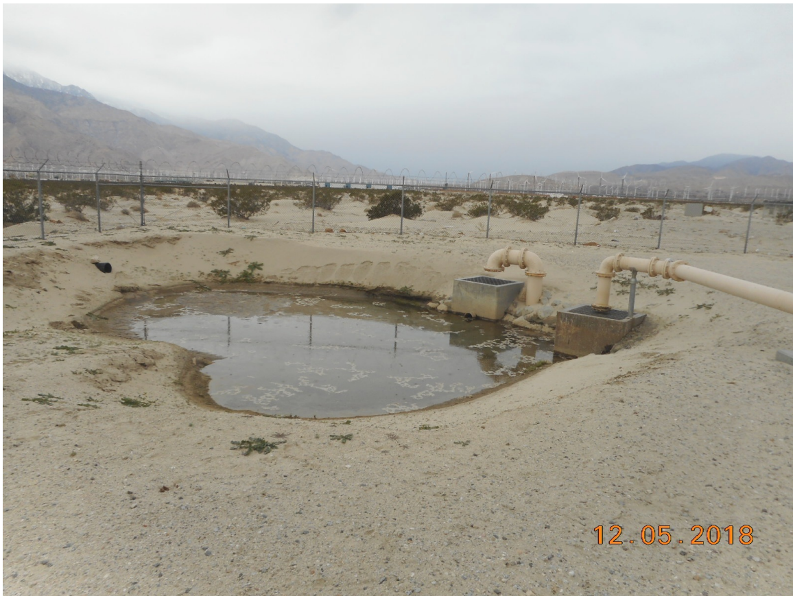
Photo 19 - View to the west-southwest, showing the drainage pond in the southwest portion of the Well No. 33 compound. The purge line for Well No. 33, typically employed when the well first begins pumping, is shown to the far right. The other pipe shown, emerging from the ground, is associated with the suction reservoir.
