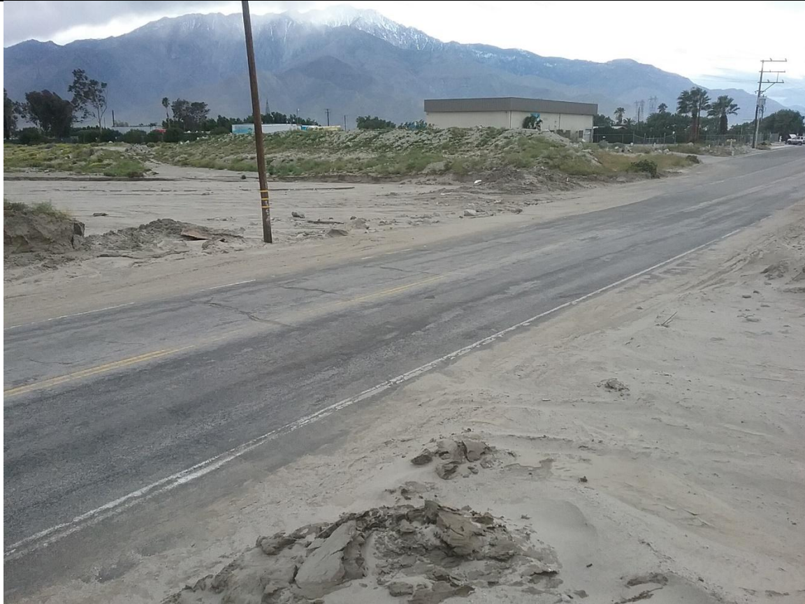
Photo 12. Looking southwest at where the proposed sewer pipeline alignment within Dillon Road crosses Mission Creek.
