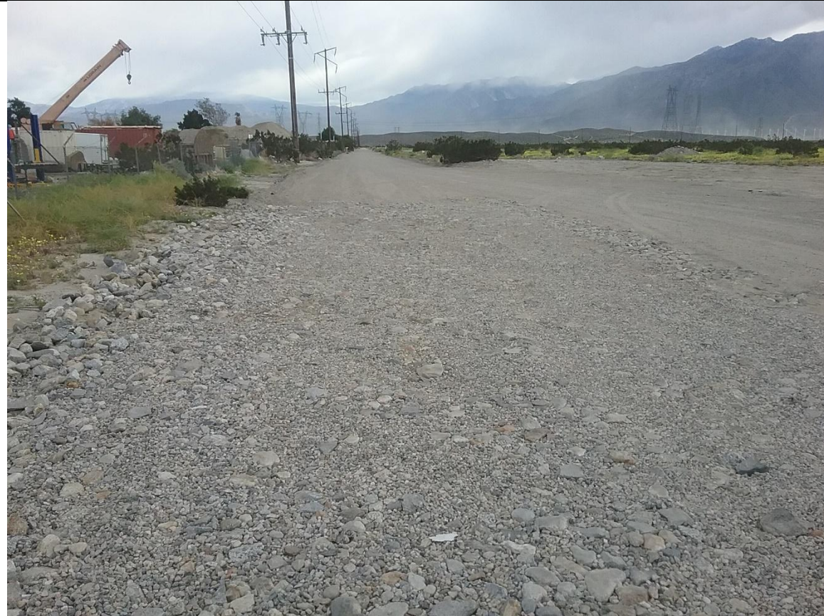
Photo 10. Looking south along the proposed sewer pipeline alignment within Little Morongo Road from the corner of Little Morongo Road and Dillon Road.
