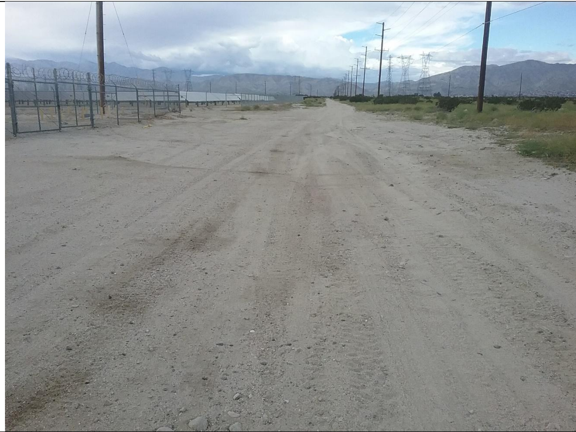
Photo 9. Looking north along the proposed sewer pipeline alignment within Little Morongo Road. District's existing Well 33 site and adjacent solar development on the left.
