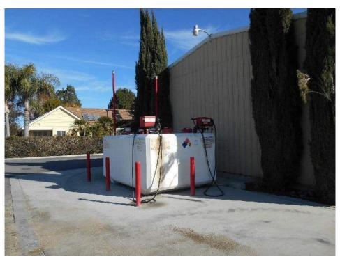
2. View of above ground concrete tank for storage of fuel.
