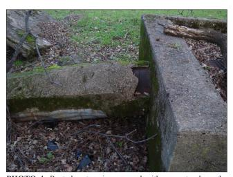
PHOTO 4: Rusted water pipe encased with concrete along the Sacramento River in the northwestern corner of the Subject Property.
