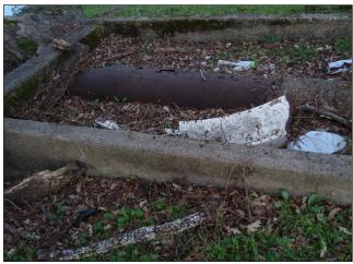
PHOTO 3: Rusted water pipe encased with concrete and scattered debris along the Sacramento River in the northwestern corner of the Subject Property.
