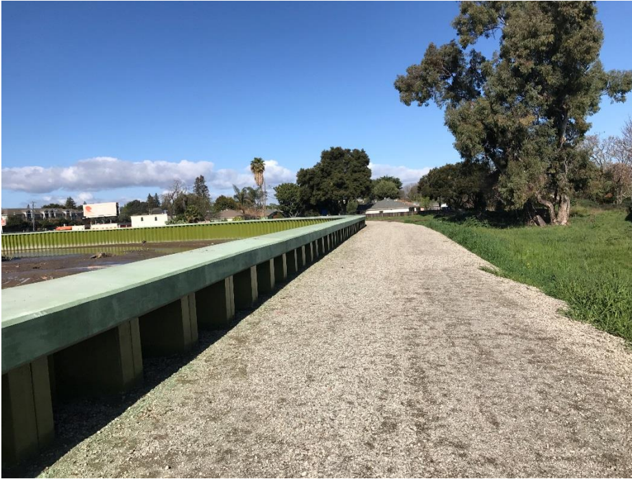
Figure 2-9. Example Sheet Pile Floodwall
