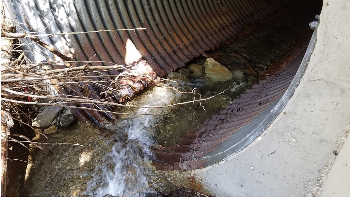
Figure 1-3 Severe Deterioration of Existing Culvert Invert
