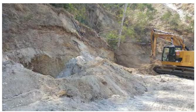
Photo 11: Excavator Pot-Holing along North-Facing Slope
