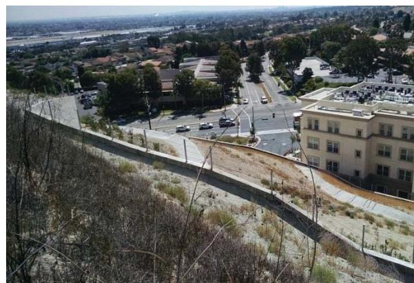
Photo 20. Facing southeast toward concrete wall where there is evidence of sheet flow that drains into a series of concrete v-ditches along southern property boundary.
