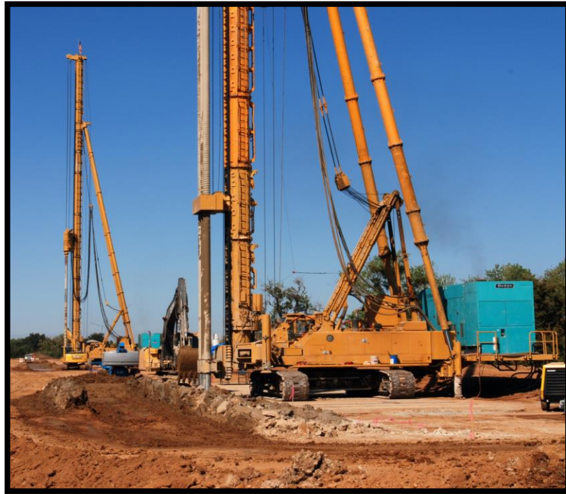
Figure 7. DMM Cutoff Wall Construction.
