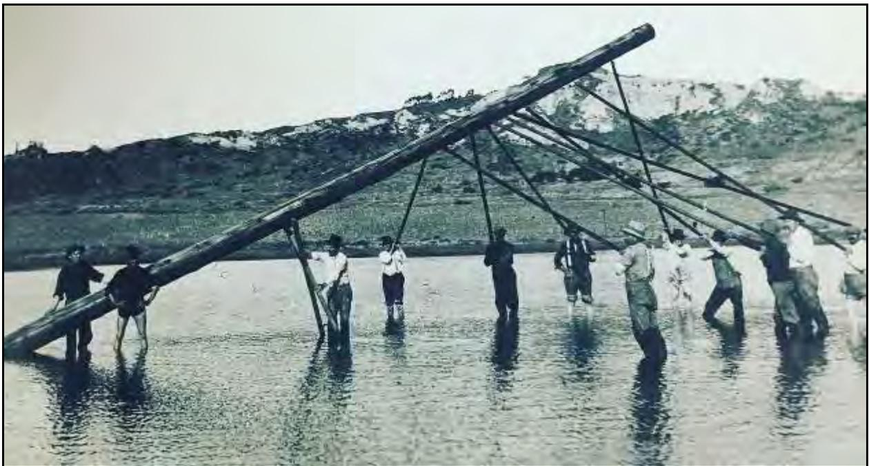
**Plate 4. Raising of an SDG&E Pole in San Dieguito Lagoon (Engstrand and Crawford 1991).**
