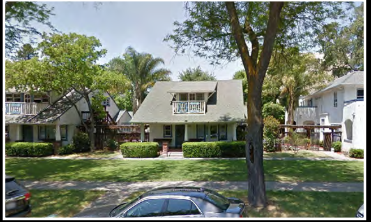
View north on First Street - Bryson House
