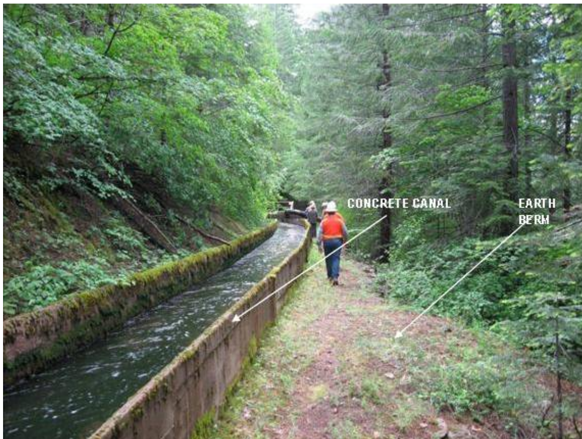
Photograph 2.2.4-1a Kilarc Main Canal – Concrete Section
