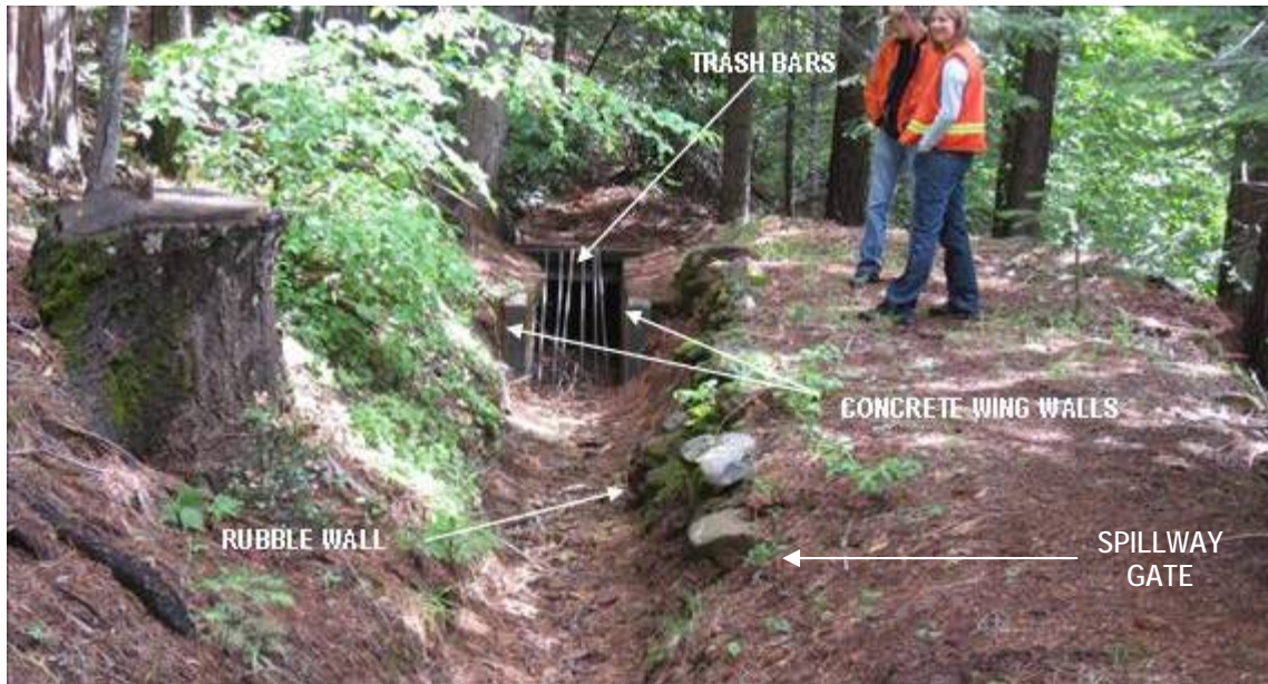
Photograph 2.2.2-1d South Canyon Creek – Canal Siphon Inlet
