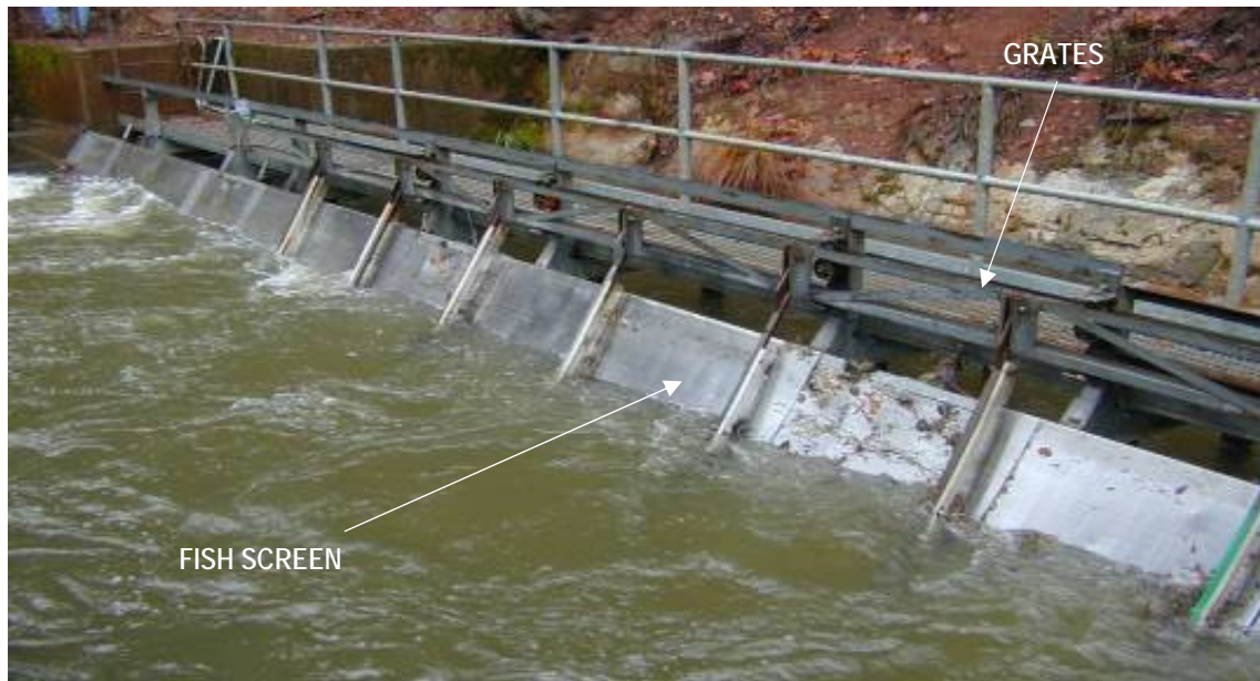
Photograph 2.3.3-1c South Cow Creek Diversion – Fish Screen Detail
