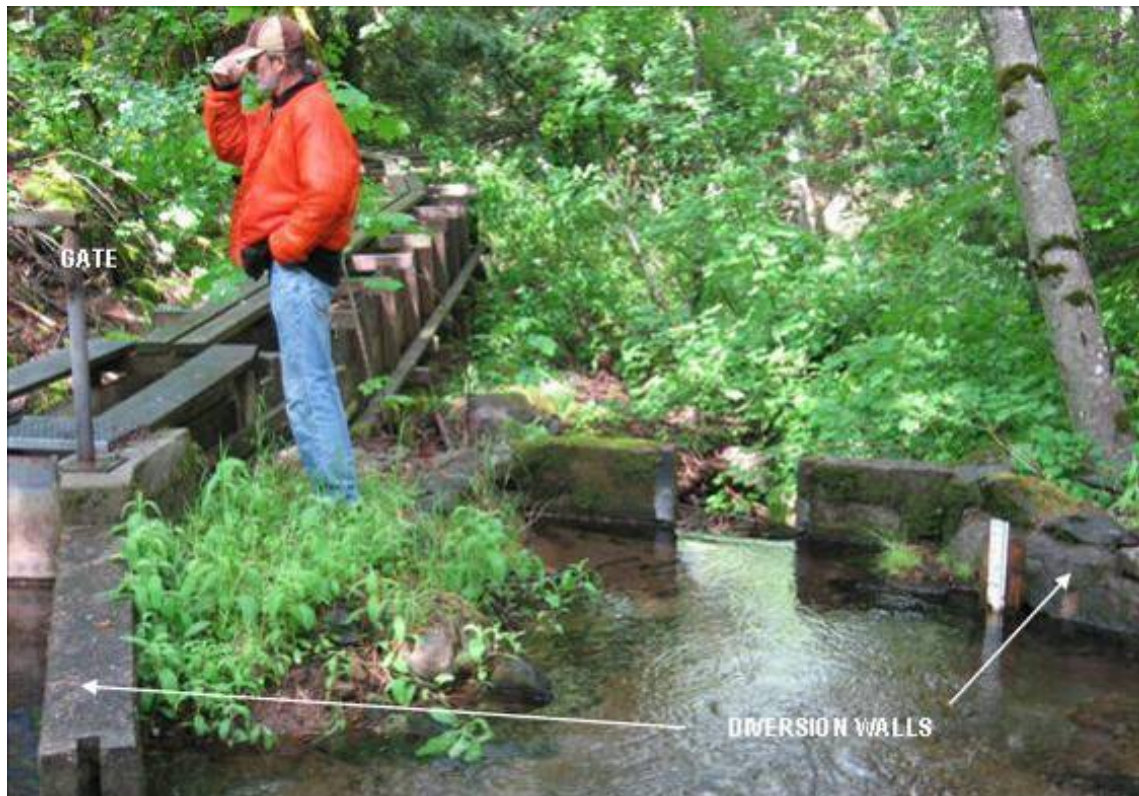
Photograph 2.2.2-1a South Canyon Creek – Diversion and Canal Inlet
