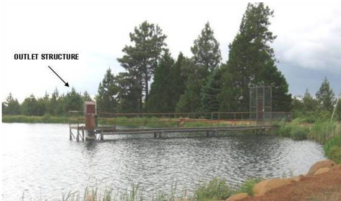
Photograph 2.2.5-1d Kilarc Forebay – Outlet Structure to Penstock
