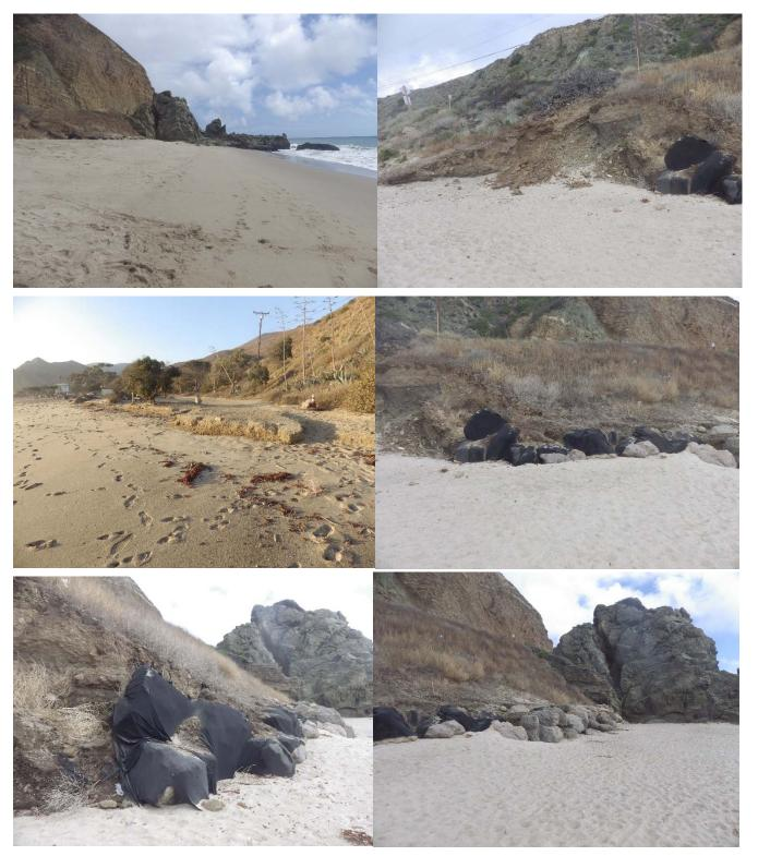
Figure A-1-3: Photos at southeast end of beach from March 2018 showing: top left entire beach with erosion escarpment in left of photo, middle left (this photo from Oct. 2017) former location of life guard structure lost during Hurricane Marie, bottom left exposed geotextile and mesh in erosion escarpment. Top to bottom on right is a pan of the erosion escarpment, toe protection rock and headland.
