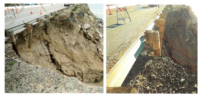
Figure 1-3: Fill slope eroded at PM 4.0 with guardrail hanging. Photo taken on 01/29/2015.
