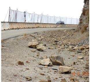
Figure 1-16: K-rail and fencing deployed within the project area. Photo taken on August 27, 2018.
