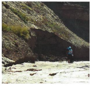
Figure 1-9: High surf causes the fill slope to erode months after reconstruction. Photo taken on 09/30/2015.
