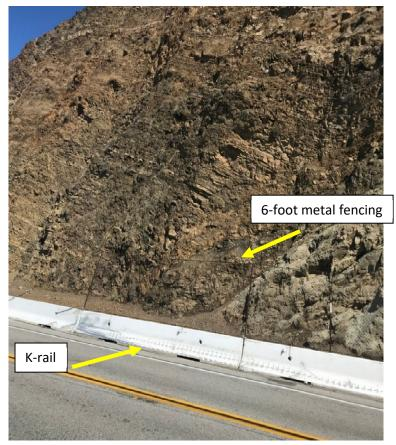
Figure 1-15: Access on the shoulder of northbound PCH through the project area is blocked with K-rail and metal fencing.
