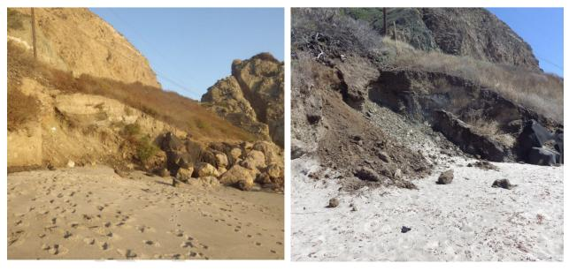
Figure 1-11: Slope on PM 4.2 in October 2017. Slope has eroded to meet the rock slope protection wall at the toe of the slope.
