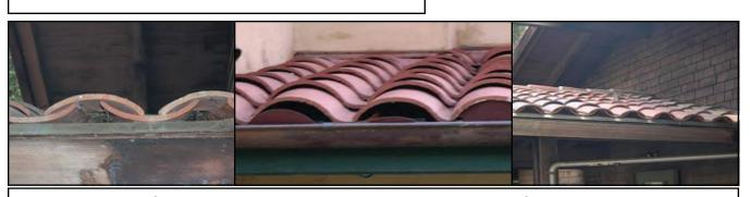
Breaches in roof tiles have allowed embers to enter and spread fire through out the home
