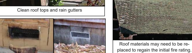
Burning embers were blown through this vent screen and a fire started in the crawl space of this home.
