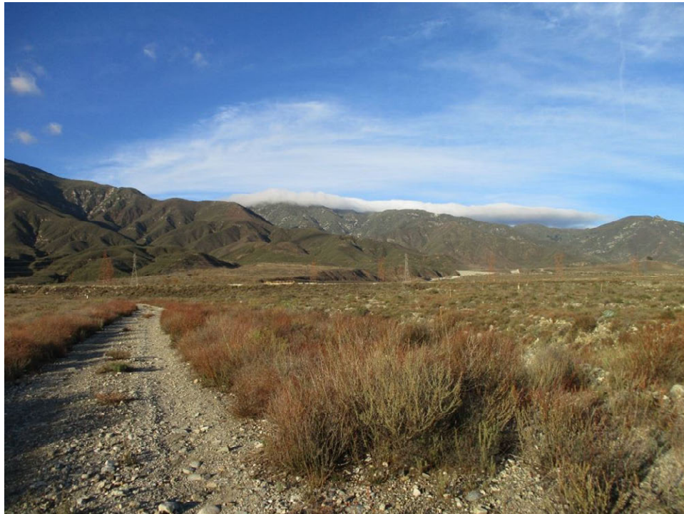
Figure 20 Looking north toward 1-602-5A Day Creek Spreading Grounds Levee (IMG_1643)
