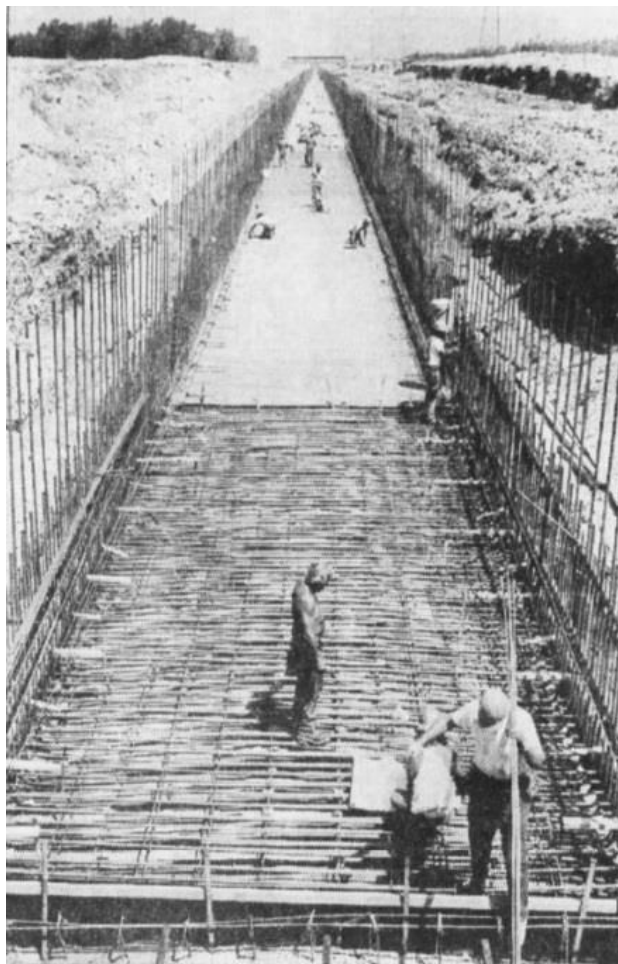
Figure 12 Fontana Steelworkers work Day Creek Flood Control Channel (SBC Sun 1989)
