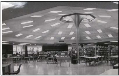
Figure 9: Interior of PHL in 1978, showing the unimpeded space created by having only the one pillar of the roof system. (Source: PHL archives)
