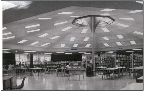
Interior of PHL in 1978, showing the unimpeded space created by having only the one pillar of the roof system. (Source: PHL archives)
