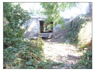
**Photo 1.** Looking upstream at the South Terrace Road culvert crossing. Note the significant drop in bed elevation at the culvert and steep streambanks bounding the channel (*September 2010*).
