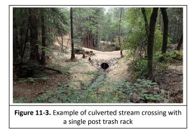
Secondary Structures at Stream Crossings. Secondary structures installed at stream crossings include downspouts and trash racks to support culvert function, and rock armor to buttress and/or reduce erosion of steep fill-slopes (Figure 11-3 and Figure 11-4). See Appendix L, typical drawings 1c, 3, and 4 for further description.
