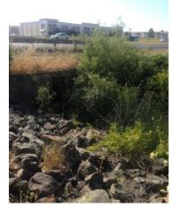
Photo 25: Vegetation blocking downstream box culvert on Sheehy Creek
