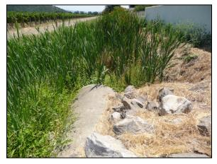
**Photo 1.** Looking downstream from Finnell Road. Dense emergent vegetation occludes the culvert at this crossing (*August 4, 2010*).
