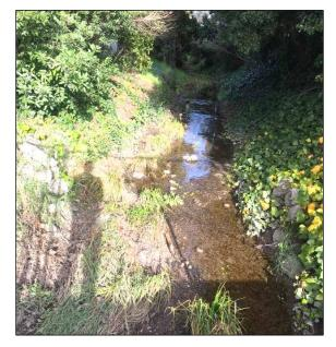
**Photo 1.** Upstream of Donaldson Way the channel supports invasive vegetation covering rock slope protection along the banks (*March 2018*).
