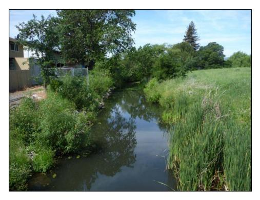
Photo 3: Reach 1 looking upstream showing channel roughness. n=0.030-0.040
