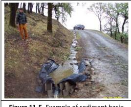
Figure 11-5. Example of sediment basin adjacent to roadway
