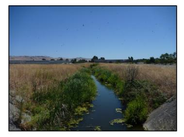
**Photo 5-3:** Fagan Creek maintenance reach, looking upstream from the inlet of the runway culvert, showing channel roughness.
