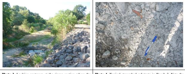
**Photo 3.** Looking upstream at the riprap section where the channel turns towards the west. Erosion-resistant riprap sloughed into the channel has resulted in some local bed scour and pooling (*August 4, 2010*).
