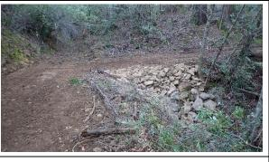
Figure 11-2. Example of an armored fill stream crossing at Simmons Canyon Creek
