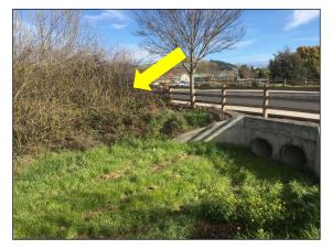
**Photo 2.** Dense willow growth (as indicated by the arrow) is causing a significant flow obstruction within the main channel upstream of Silver Oak Trail. The culverts in the foreground provide overflow capacity (*March 2018*).
