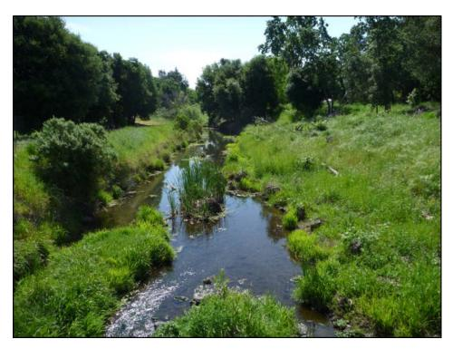
Photo 4: Reach 2 looking downstream showing channel roughness. n=0.030-0.040
