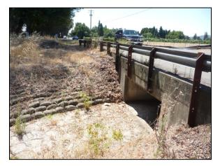
**Photo 1.** Upstream end of the SYC. A concrete box culvert passes flows (beneath Solano Ave.) from an unnamed tributary to the west into the SYC (*August 4, 2010*).
