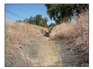
**Photo 2.** Looking downstream from the mid-point of the Solano Ditch. The channel bottom and low banks are lined with concrete. The upper banks are formed in native soils. Vegetation on the upper banks consists of non-native herbaceous species (*August 4, 2010*).
