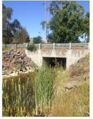
Photo 24: Box culvert with beaver dam upstream and downstream on Sheehy Creek
