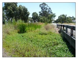
**Photo 1.** Looking downstream from upstream end of the NYC. Two concrete box culverts pass flows from the main upstream tributary into the NYC. Note the dense aquatic and emergent vegetation in the channel (*August 4, 2010*).
