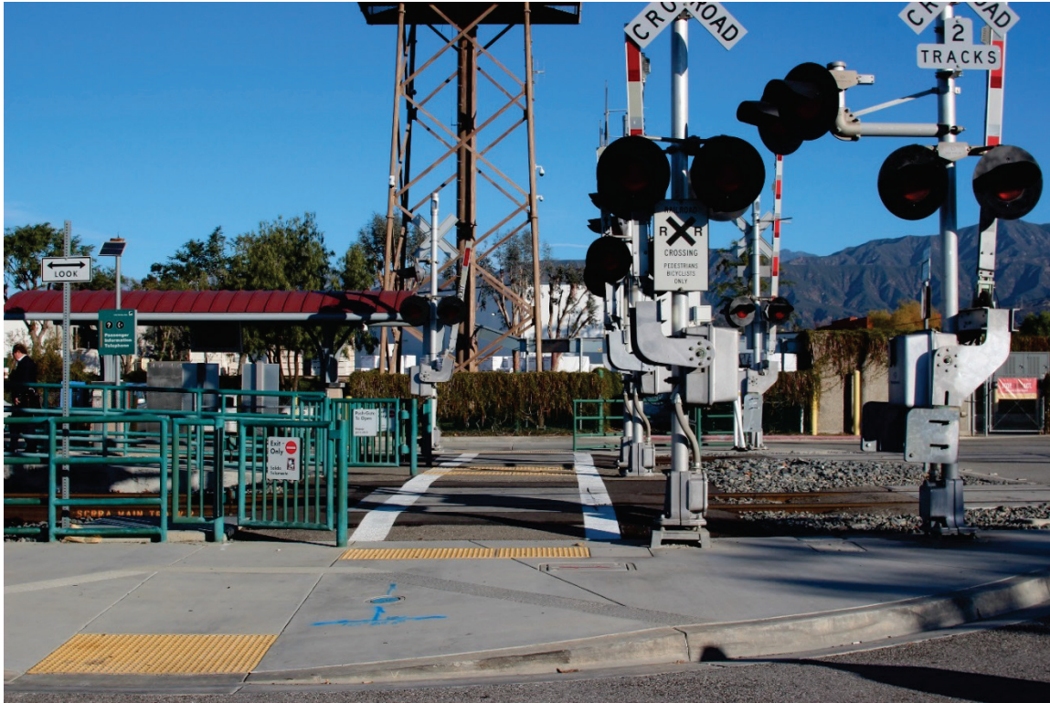
Figure 3.9-2. Existing Safety Features of the At-Grade Pedestrian Crossing at the Metrolink Pomona North Station
